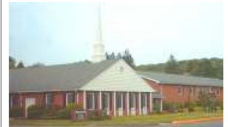
First Baptist - corner of Pearl St. & Central Ave.
