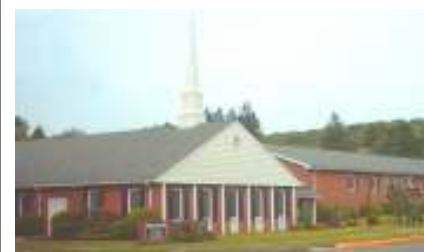
First Baptist - corner of Pearl St. & Central Ave.
