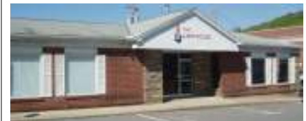
“The Lighthouse” Youth Ministry Building - Crafton Street
