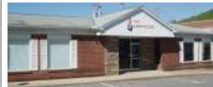
"The Lighthouse" Youth Ministry Building - Crafton Street
